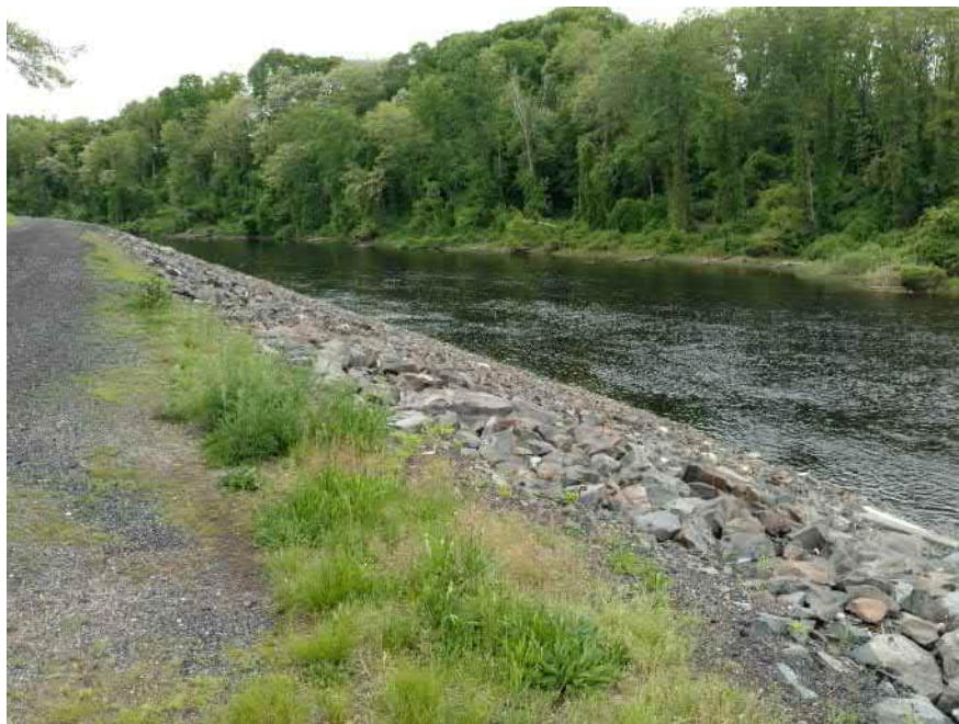
View of the Facemate Property Fill Area along the Chicopee river—facing south
