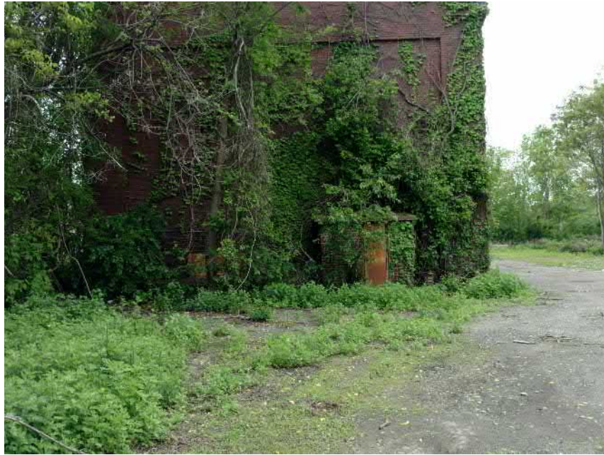
View of the existing warehouse on the Facemate Property Fill Area—facing south
