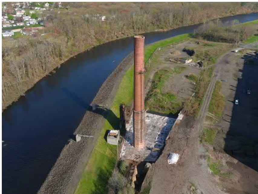
View of the Uniroyal Property Fill Area and Intake Abandonment Area—facing north
