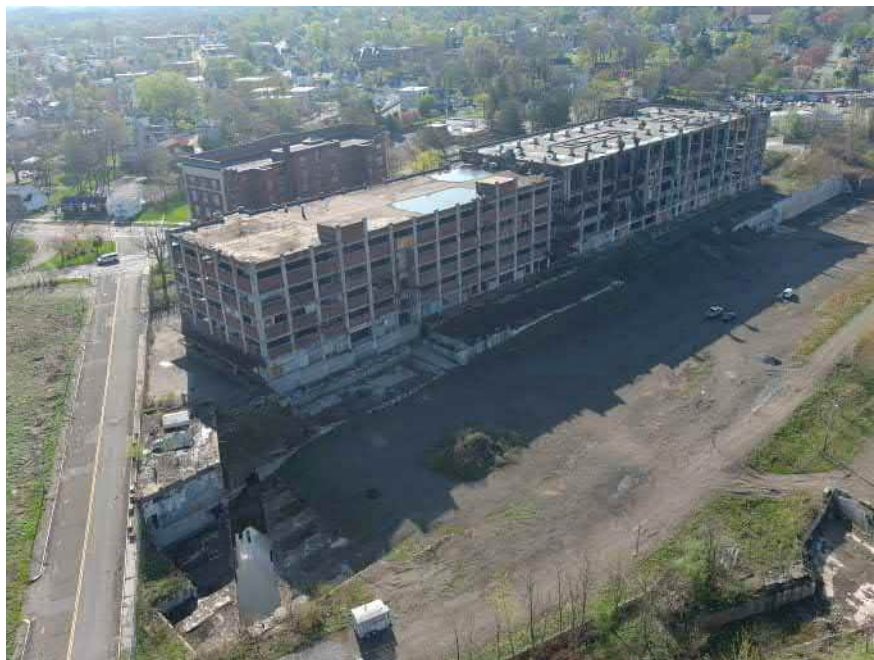
View of the Fisk Rubber Company Office buildings—facing southeast
