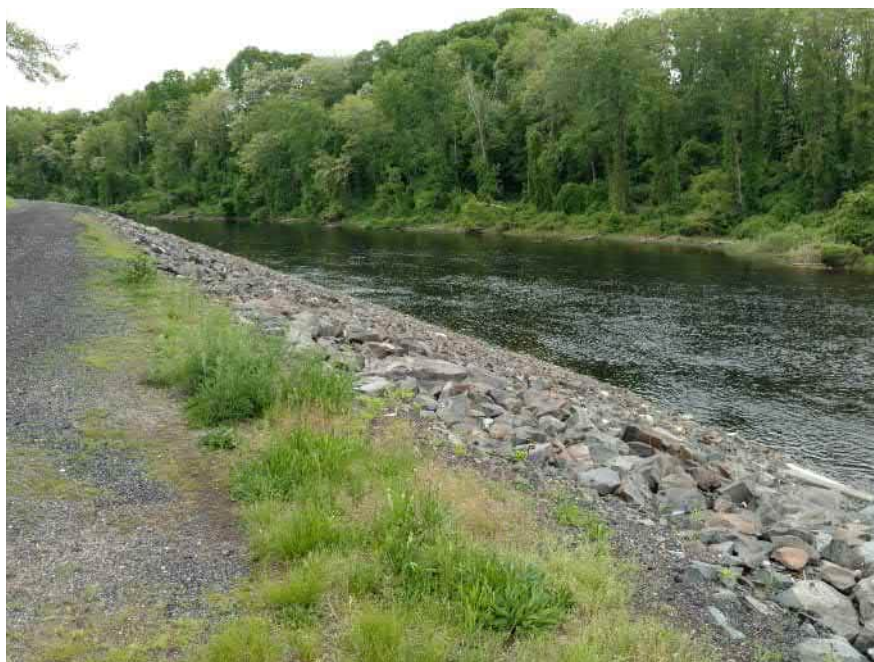
View of the Facemate Property Fill Area along the Chicopee river—facing south
