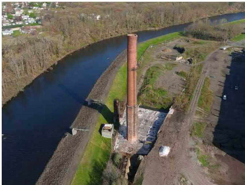
View of the Uniroyal Property Fill Area and Intake Abandonment Area—facing north
