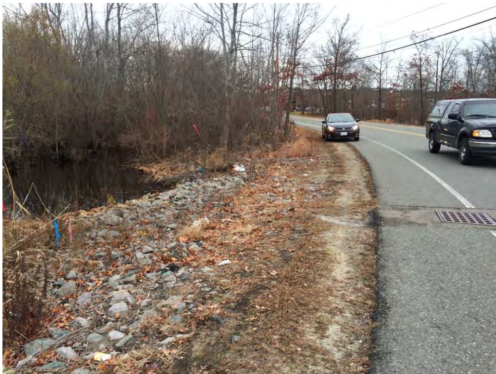
Wetlands at Existing Edge of Pavement (Sta. 44+25± LT)
