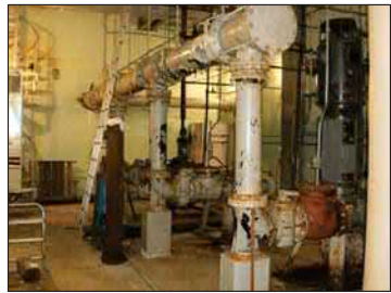
PHOTO 4 PUMP LEVEL EXISTING CONDITIONS
