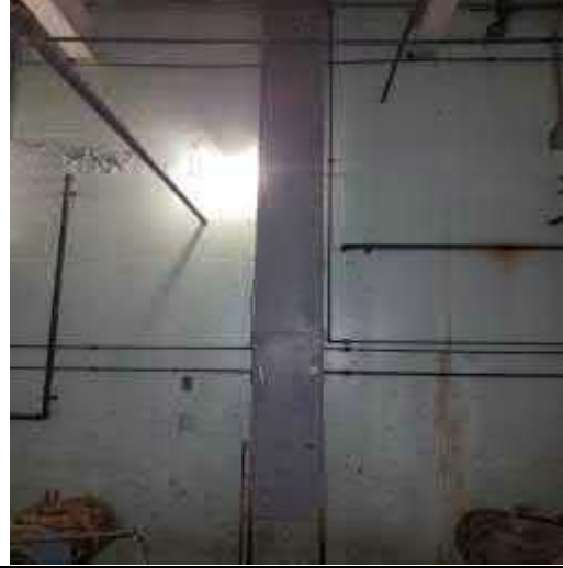
Gray duct paint
