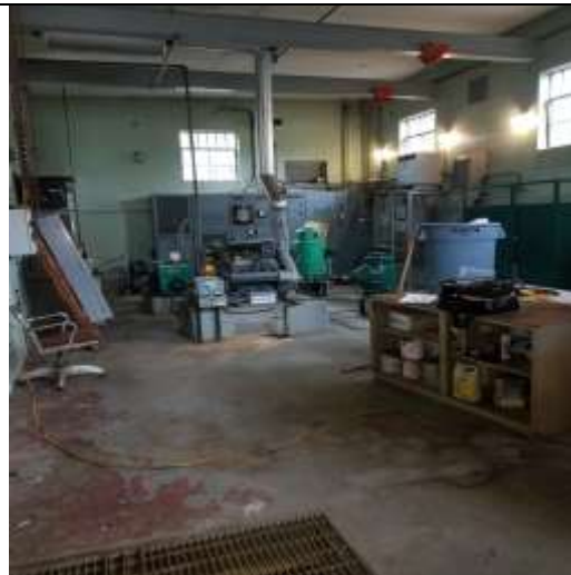
Floor 1 floor paint & general view
