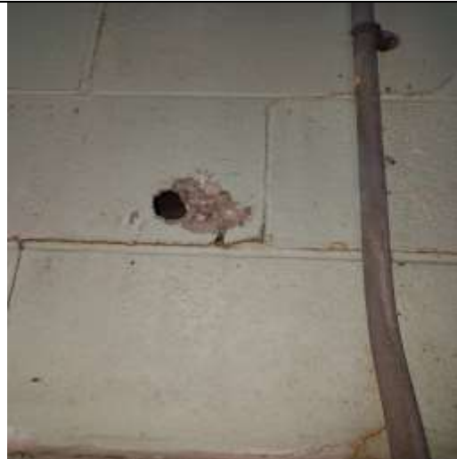
Main level cinderblock, no fillers observed
