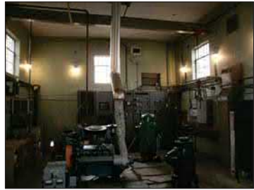
PHOTO 3 MAIN FLOOR EXISTING CONDITIONS
