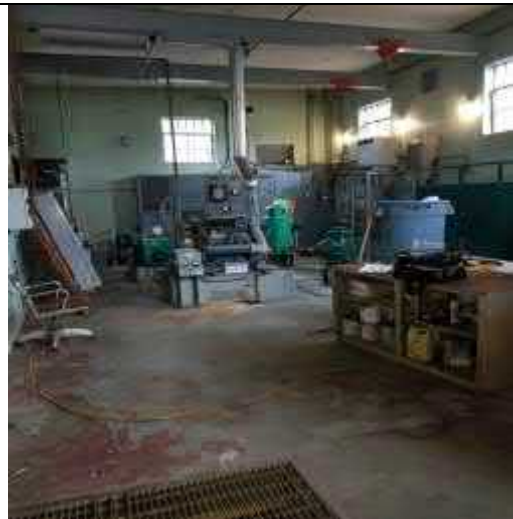
Floor 1 floor paint & general view
