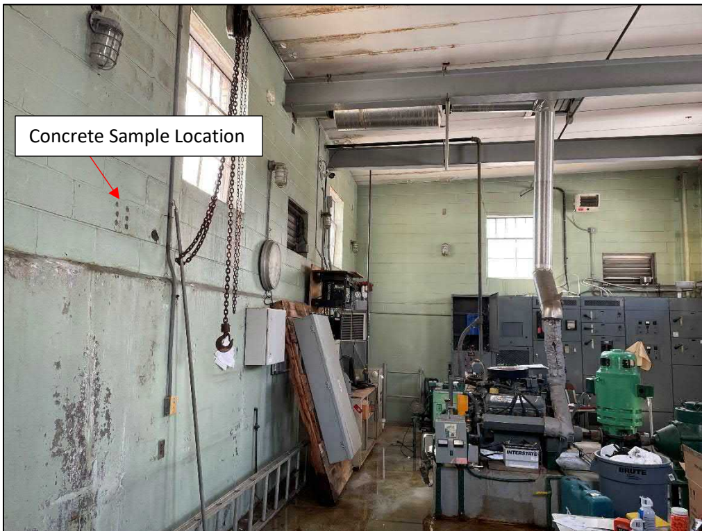
Green paint on interior walls, upper level
