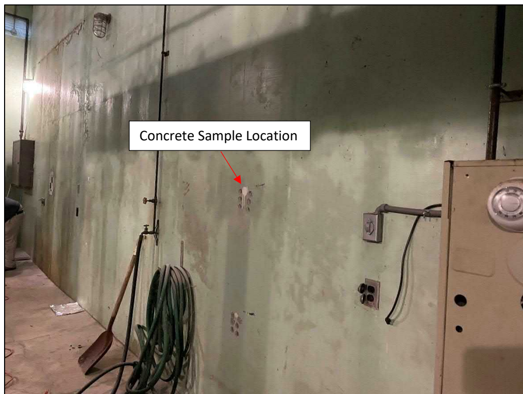
Green paint on interior walls, lower level
