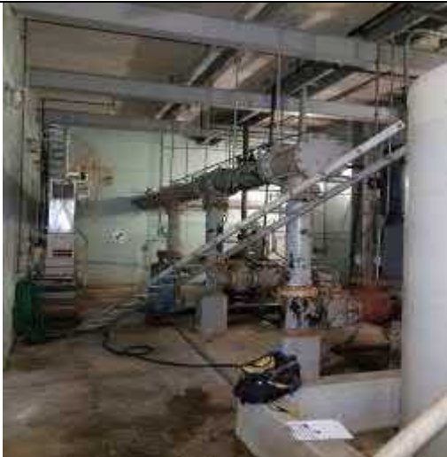
Basement general view
