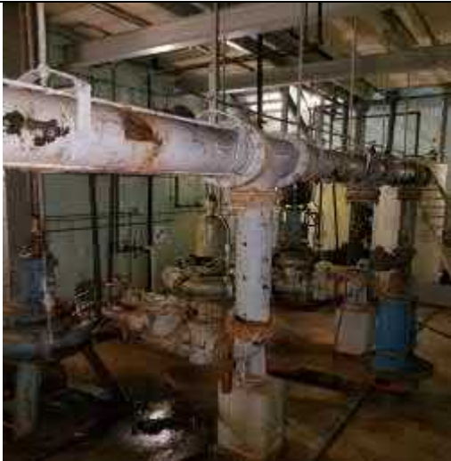
Gray pipe paint
