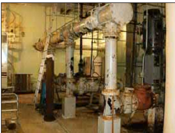
PHOTO 4 PUMP LEVEL EXISTING CONDITIONS
