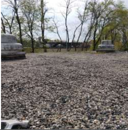
Tar & gravel roof, asbestos
