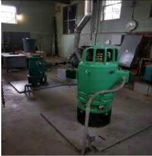
Floor 1 green motor paint
