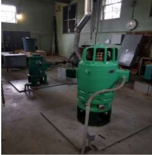
Floor 1 green motor paint
