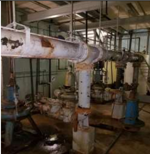
Gray pipe paint
