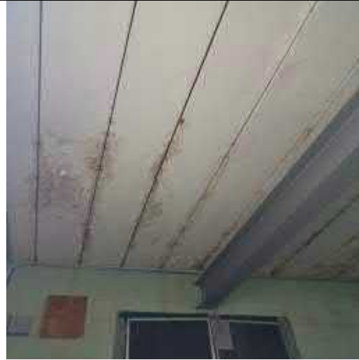
Floor 1 white painted ceiling
