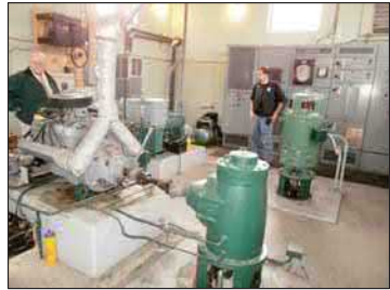
PHOTO 2 MAIN FLOOR EXISTING CONDITIONS
