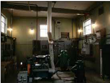
PHOTO 3 MAIN FLOOR EXISTING CONDITIONS
