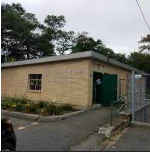
Pump Station view
