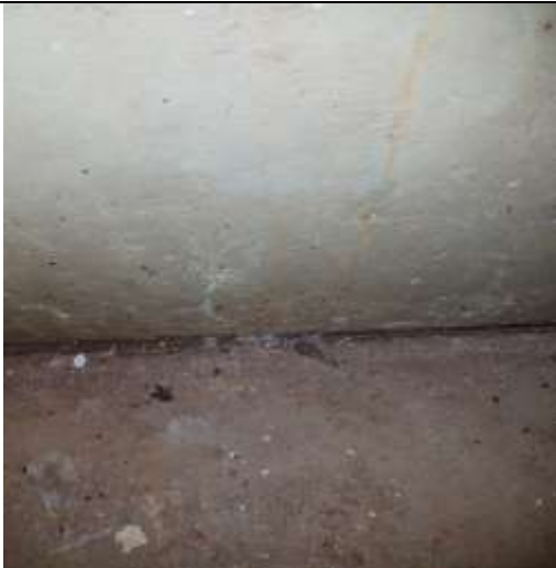
Wall seam sealer lower level outer wall
