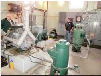
PHOTO 2 MAIN FLOOR EXISTING CONDITIONS
