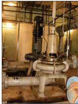
PHOTO 5 PUMP LEVEL EXISTING CONDITIONS
