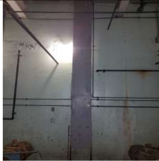
Gray duct paint
