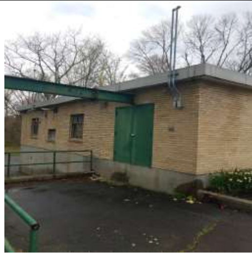
Side dock entrance
