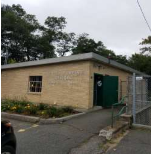
Pump Station view
