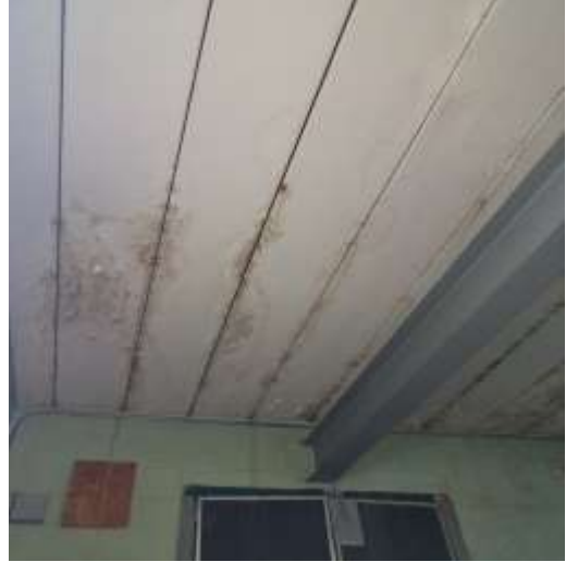
Floor 1 white painted ceiling
