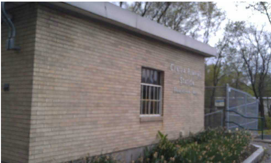
Worcester Road Pump Station
