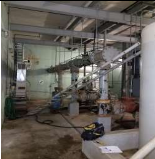
Basement general view
