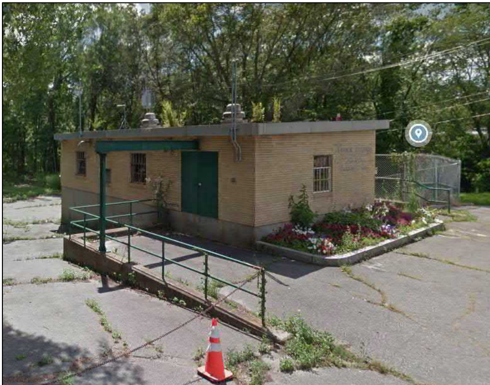
Site building exterior, looking southwest
