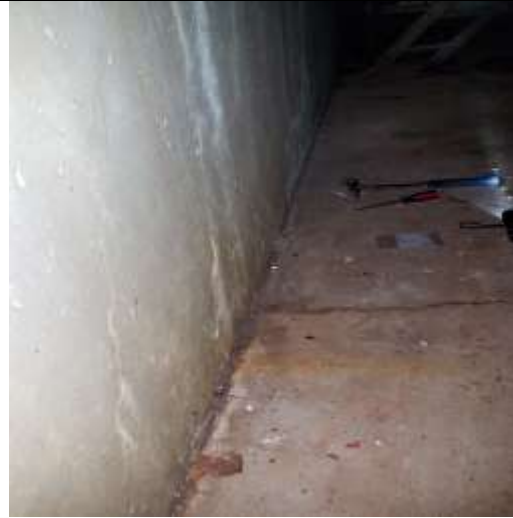
Wall seam sealer lower level outer wall
