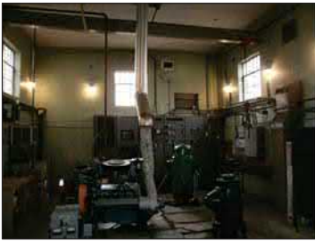
PHOTO 3 MAIN FLOOR EXISTING CONDITIONS
