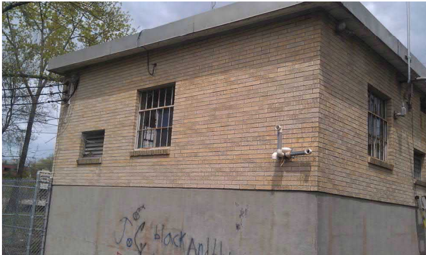
ACM – Window and Louvered Vent Caulking
