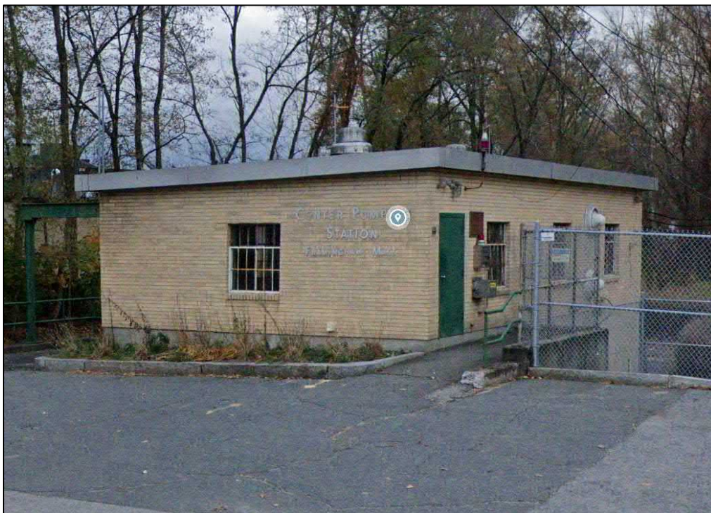
Site building exterior, looking southeast
