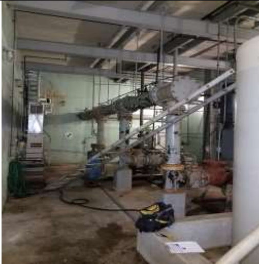
Basement general view
