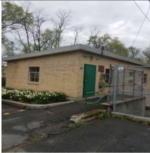
Front main entrance
