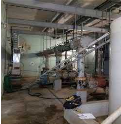
Basement general view
