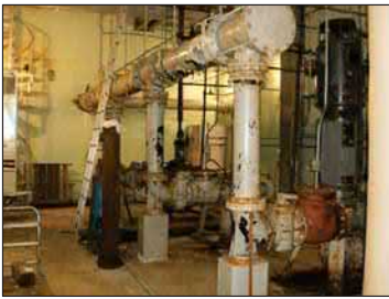
PHOTO 4 PUMP LEVEL EXISTING CONDITIONS
