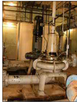
PHOTO 5 PUMP LEVEL EXISTING CONDITIONS
