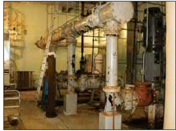
PHOTO 4 PUMP LEVEL EXISTING CONDITIONS
