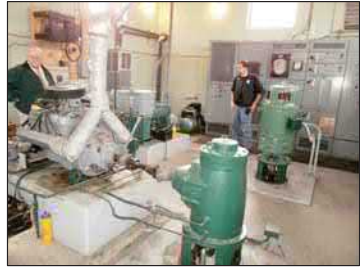
PHOTO 2 MAIN FLOOR EXISTING CONDITIONS
