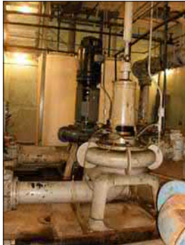
PHOTO 5 PUMP LEVEL EXISTING CONDITIONS
