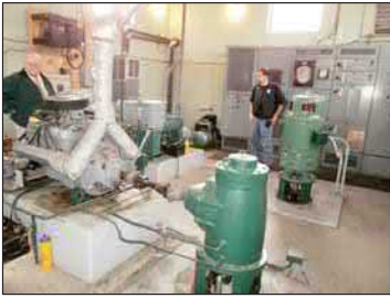
PHOTO 2 MAIN FLOOR EXISTING CONDITIONS
