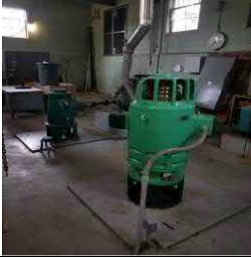
Floor 1 green motor paint
