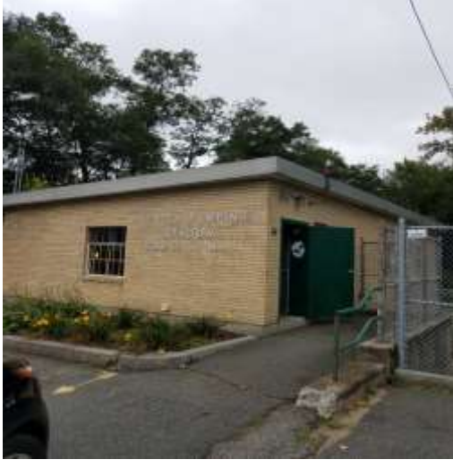
Pump Station view
