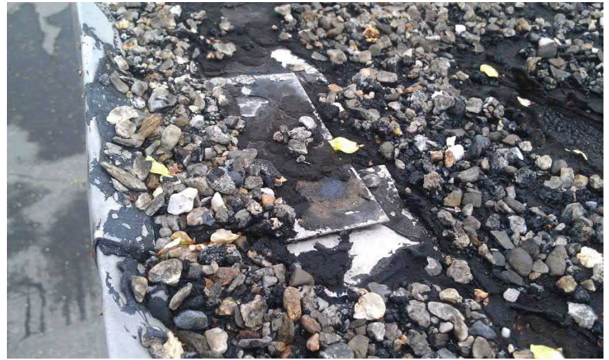
Roofing with Trace Asbestos
