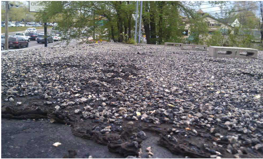
Roofing with Trace Asbestos
