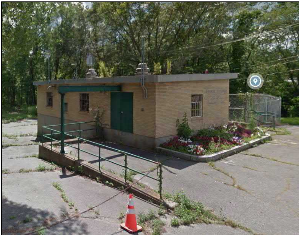
Site building exterior, looking southwest
