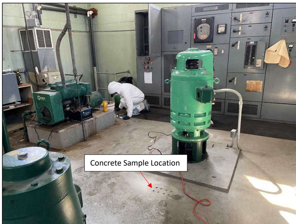
Gray paint on floor and green paint on equipment, upper level
