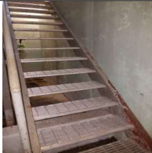
Gray stair system paint
