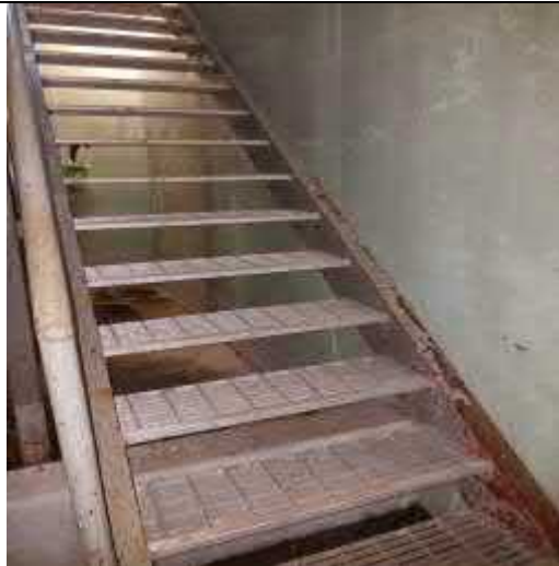
Gray stair system paint
