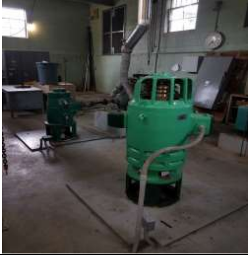
Floor 1 green motor paint
