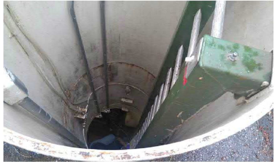
Kittredge Road Pump Station Access
