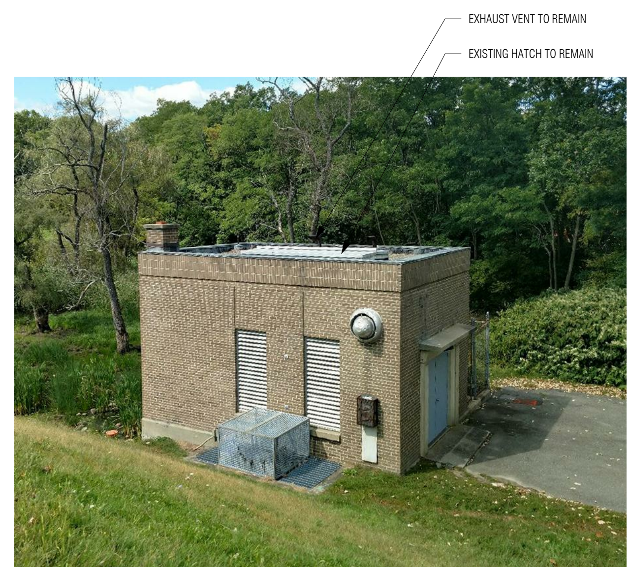
3 PHOTO - EXISTING SAXONVILLE PUMP STATION 3" = 1'-0"
