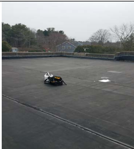
View of roof
