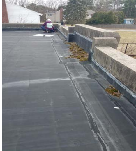
Front view of roof wall
