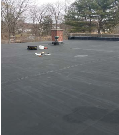
View of roof
