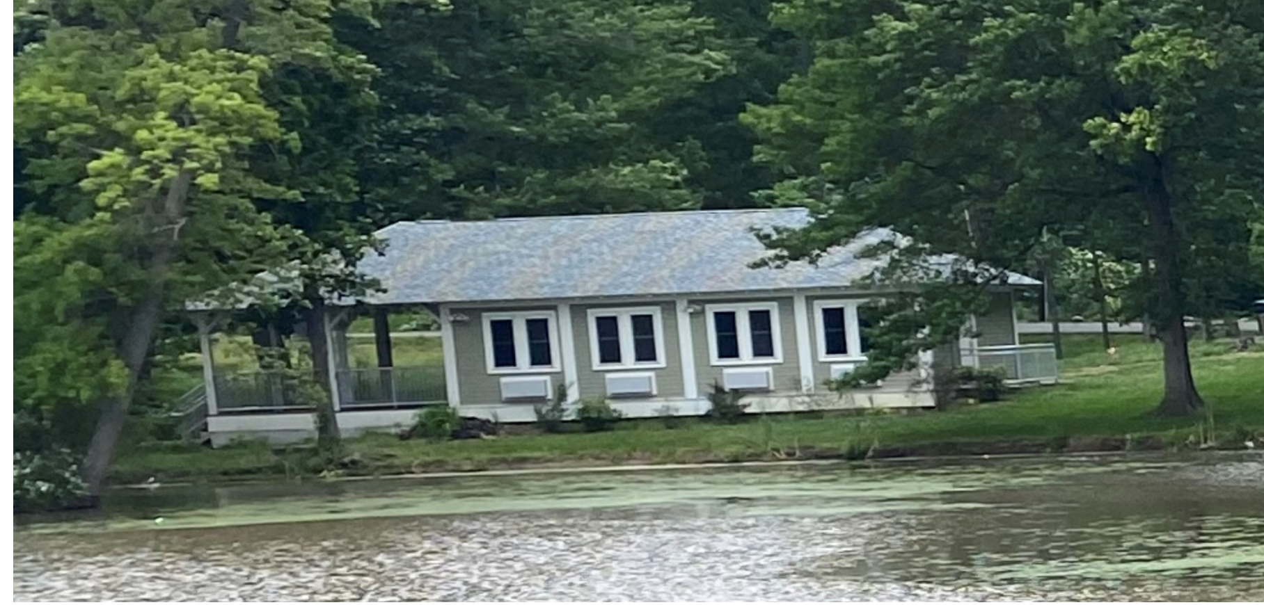
Existing Building Near Proposed Pump House Scale: NTS
