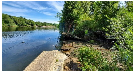
View of existing river wall – looking south
