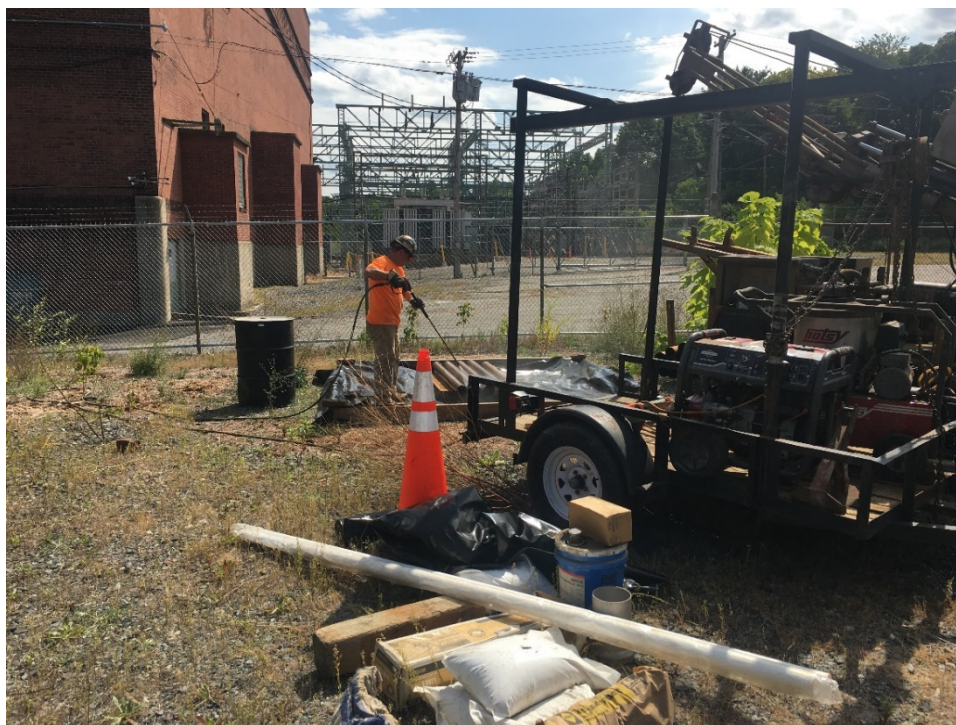
Steam Cleaning Set up on the Tidewater Site
