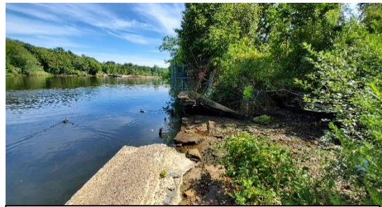
View of existing river wall – looking south
