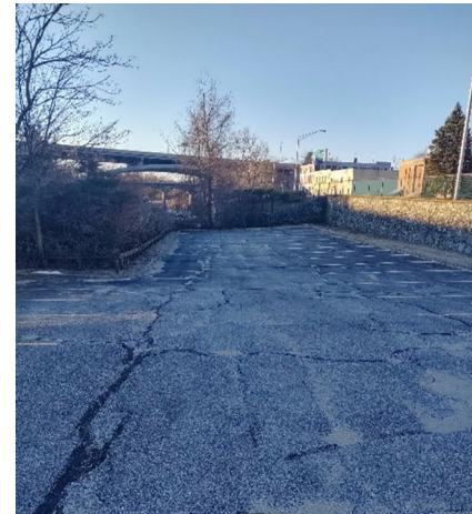
View of Parcel 584 Retaining Wall – Looking south
