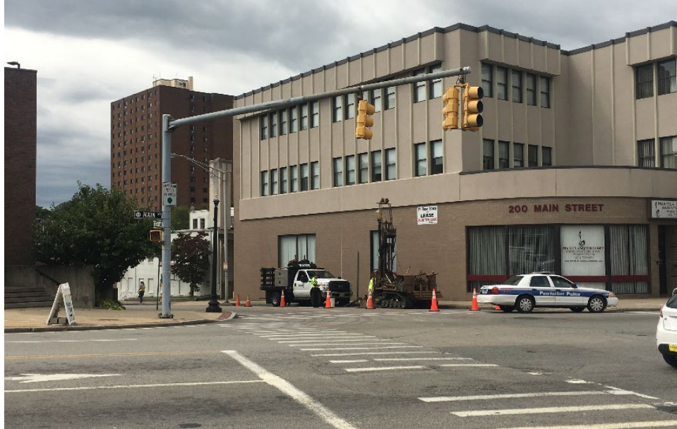
Drilling Test Boring B-8 at the Intersection of South Main St. and Roosevelt Ave. Ext.
