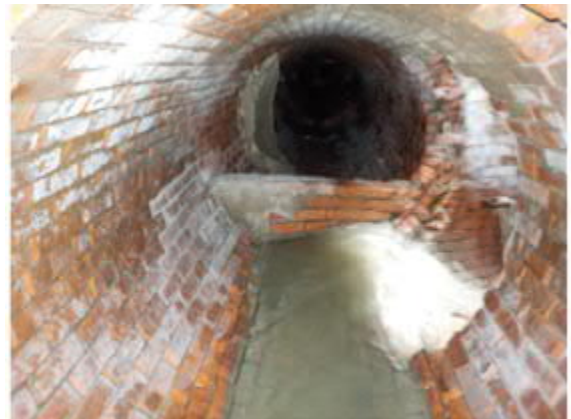
Photograph of OF-210: OF-211 pipe is to the right and brick weir is the regulator
