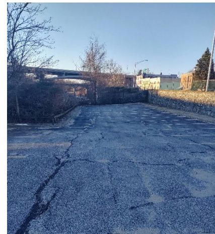
View of Parcel 584 Retaining Wall – Looking south
