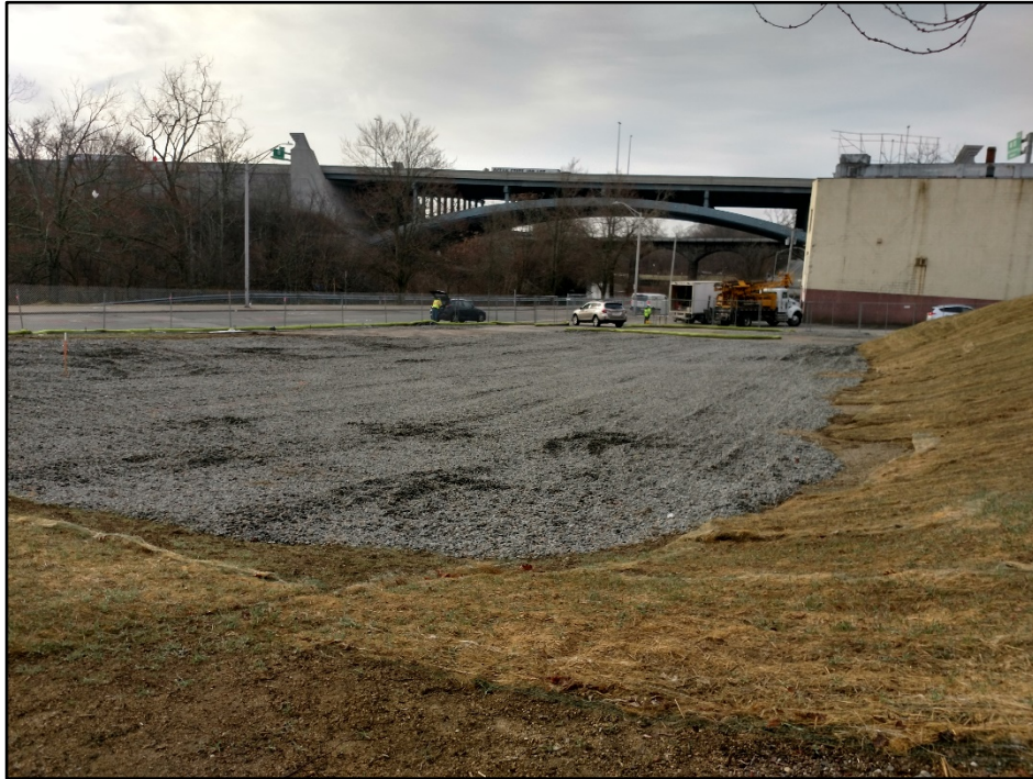
Photograph 1: Northwest corner facing Southeast
