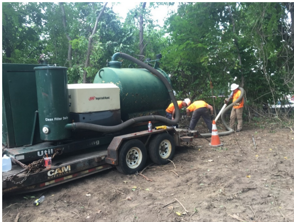
Vacuum Excavation at Test Boring B-3
