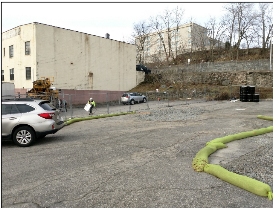
Photograph 8: Southeast side facing Southwest towards adjacent building and up slope.
