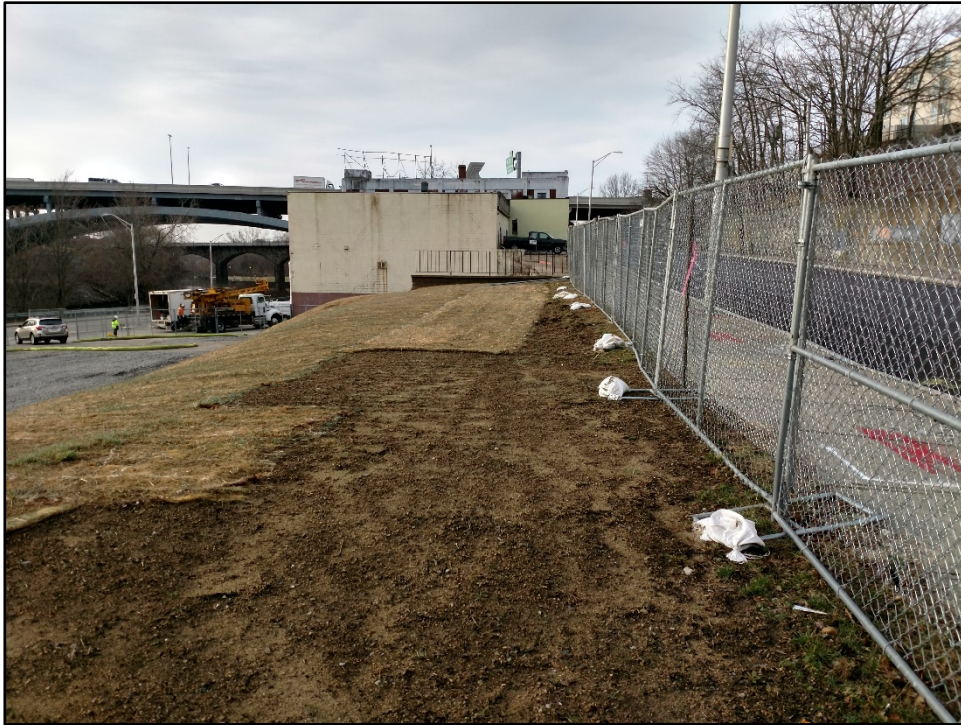
Photograph 9: Northwest corner looking South, Pleasant Street to right.
