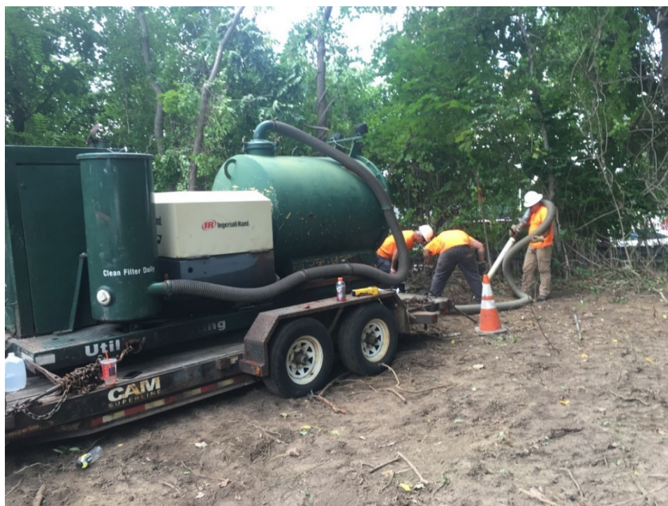
Vacuum Excavation at Test Boring B-3
