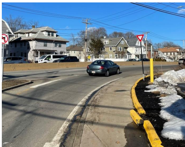
Image 3: Substandard Yield Sign and lack of pavement markings
