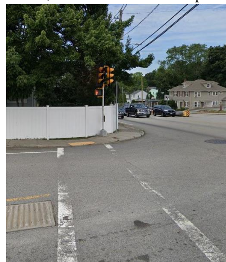
Image 2: Fence Blocks Visibility on the Southwest Corner
