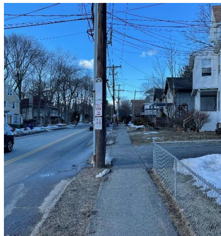
Image 4: Non-accessible bus stop on Woodward Street
