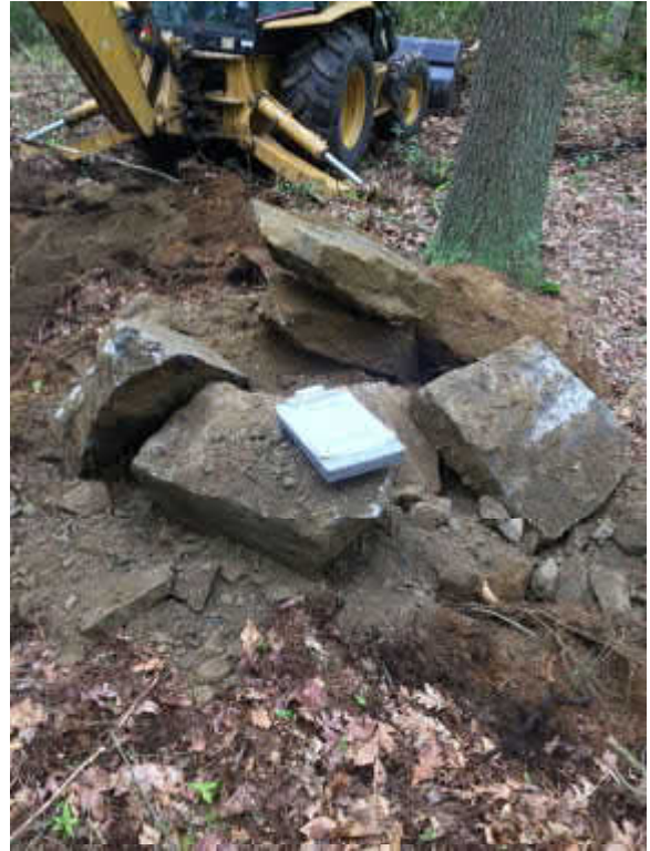
Test Pit 2 - Boulders
