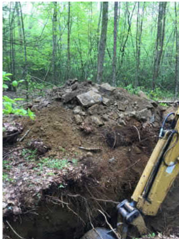
Test Pit 2 – Spoils
