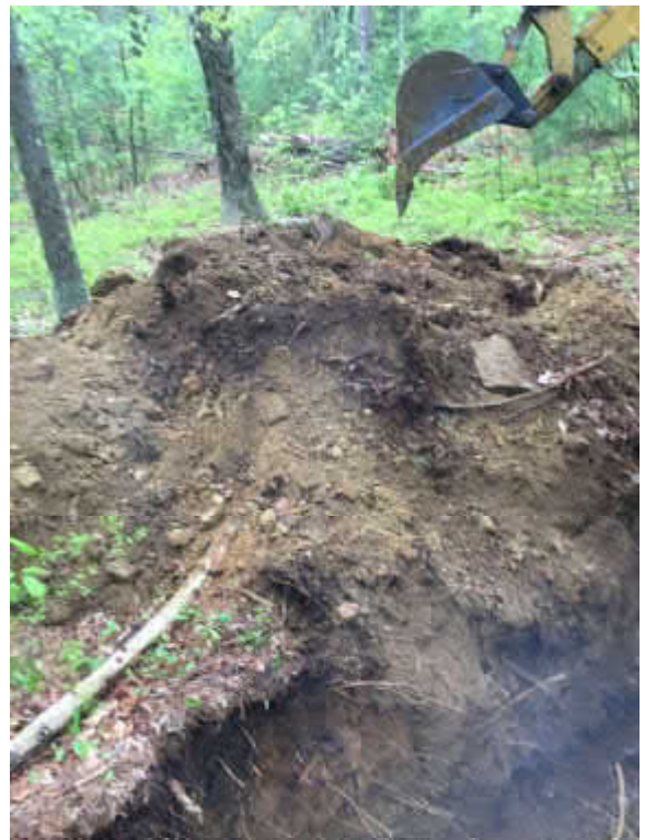
Test Pit 1 – Spoils
