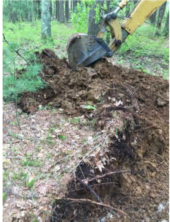
Test Pit 4 - Spoils
