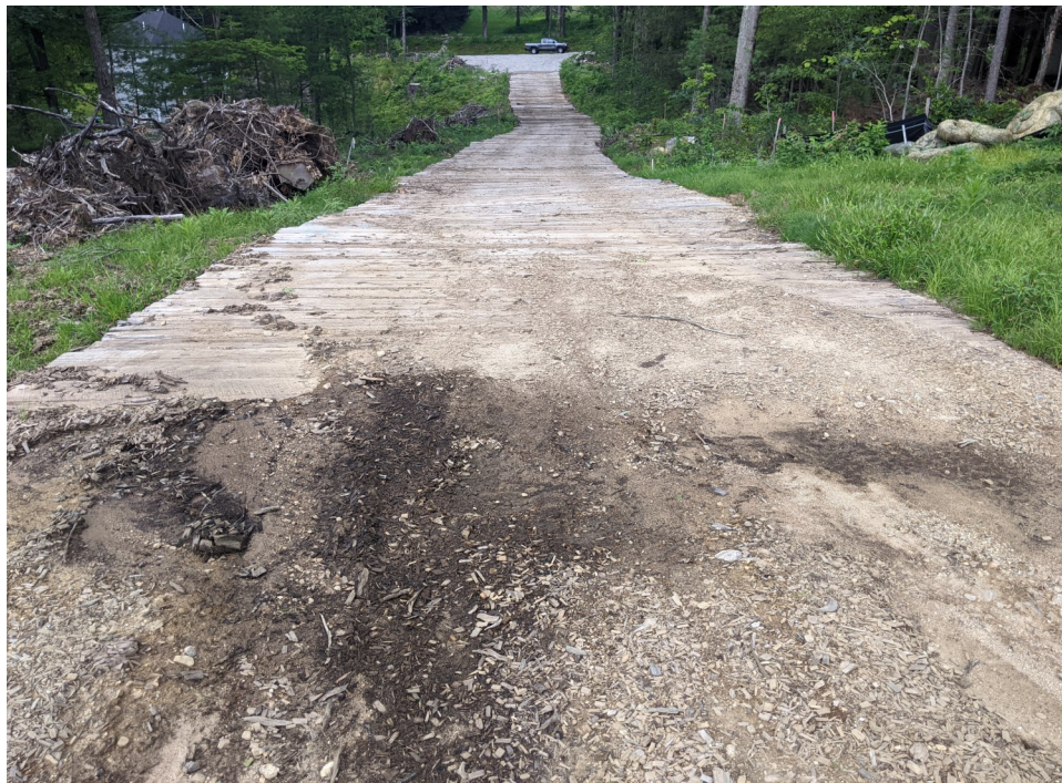
View of erosion within the access road to the north of the stockpile area—facing north.
