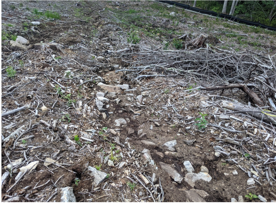
View erosion gullies beginning to form upgradient of the informal northern access road—facing northwest.
