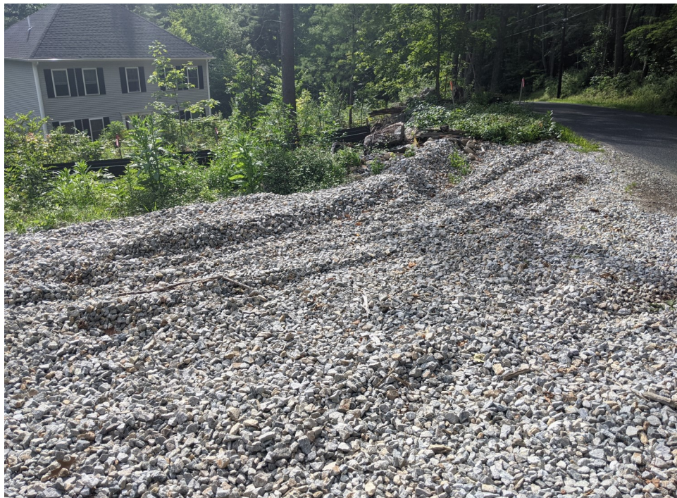
View of the stabilized construction entrance—facing west.
