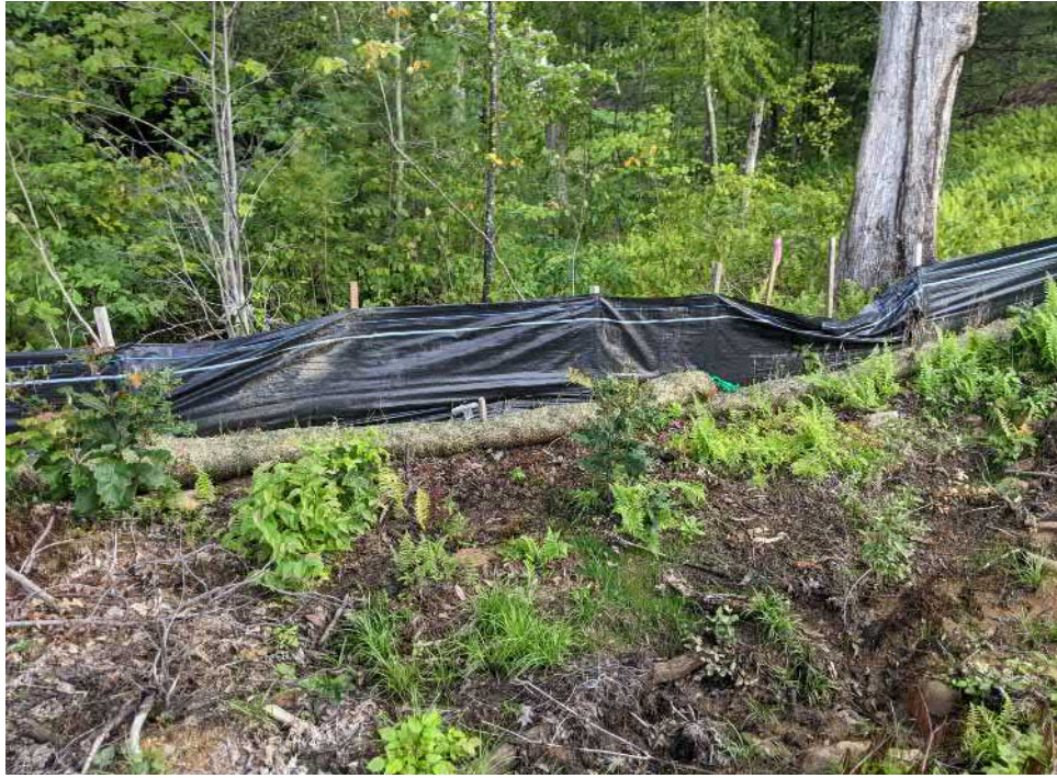
View of re-established straw wattles—facing north.
