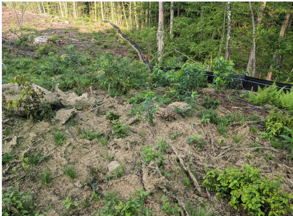
View of hydroseed applied to exposed soils to the southwest of the timber mats—facing northwest.
