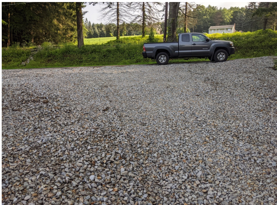
View of the recently maintained construction entrance—facing north.
