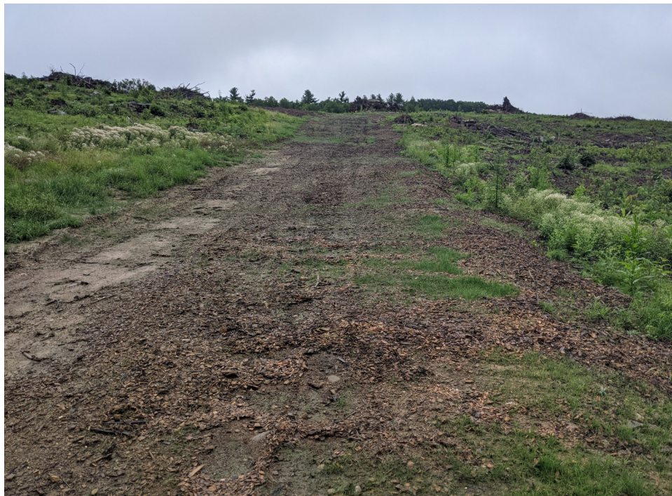
View of conditions within the access road leading to the stockpile area—facing south.
