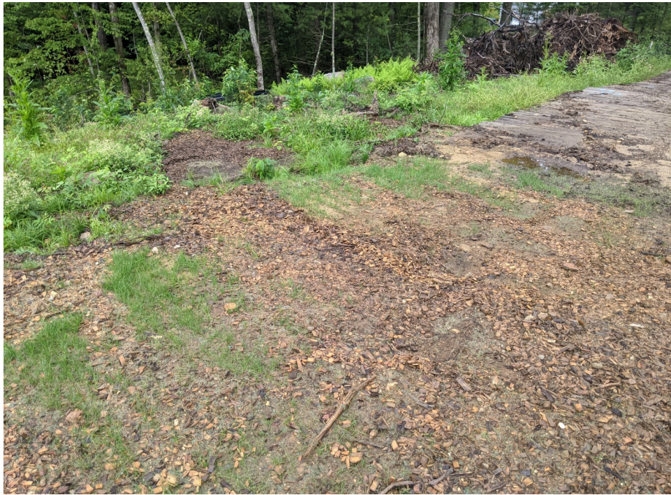
View of an area contributing runoff to the area of the former erosion control breach; note the channel forming to the left of the timber mats—facing northwest.
