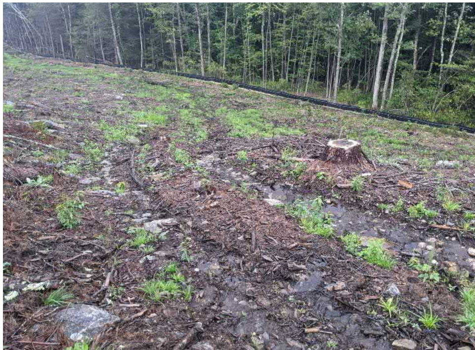
View of erosion channels at the location of the informal access path along the northern limits of work—facing northwest.
