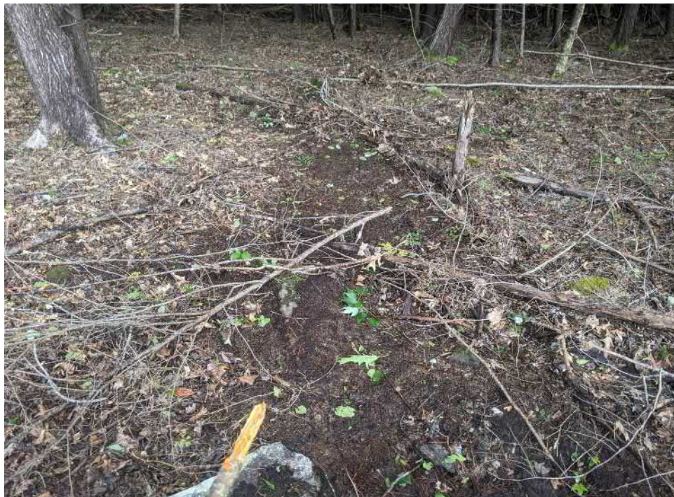
View of scour beyond the northern limits of work resulting from runoff undercutting the siltation fencing (Discharge 2)—facing north.
