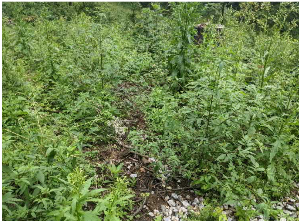
View of scour associated with the exposed soils at the construction entrance; this scour is confined to the limits of work—facing southwest.
