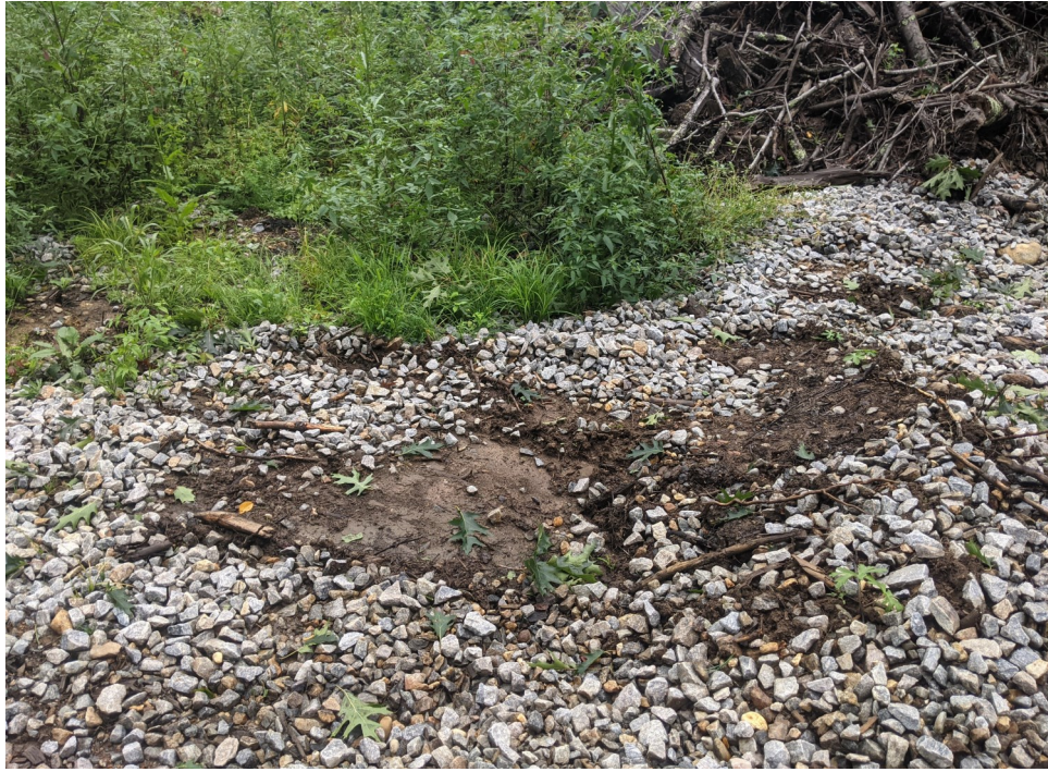
View of exposed soils along the west side of the stabilized construction entrance—facing west.
