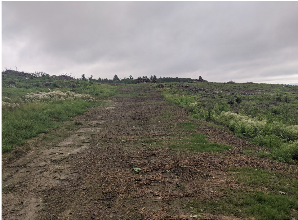
View of the earthen access road—facing south.
