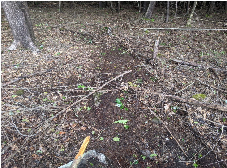
View of scour just beyond the northern limits of work due to runoff undercutting the siltation fencing (Discharge 2)—facing north.
