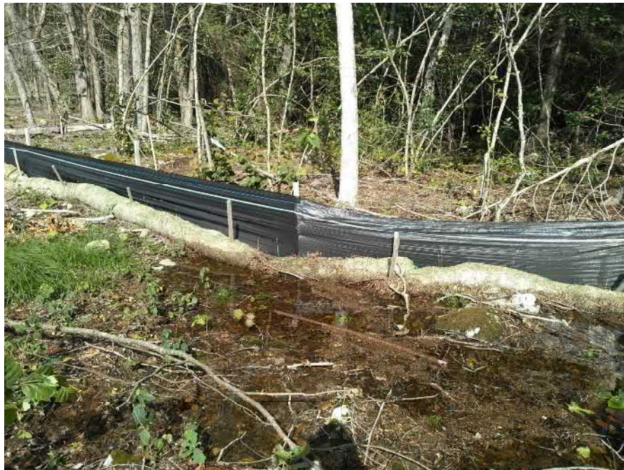
View of degraded straw wattle at southeast perimeter of Site —facing east.
