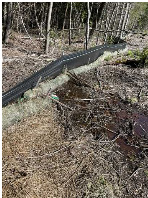
View of degraded straw wattle at southeast perimeter of Site —facing east.
