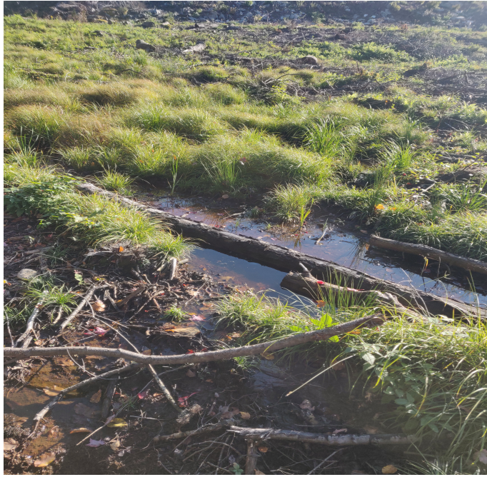
View of the water pooling in western perimeter of Site —facing east.
