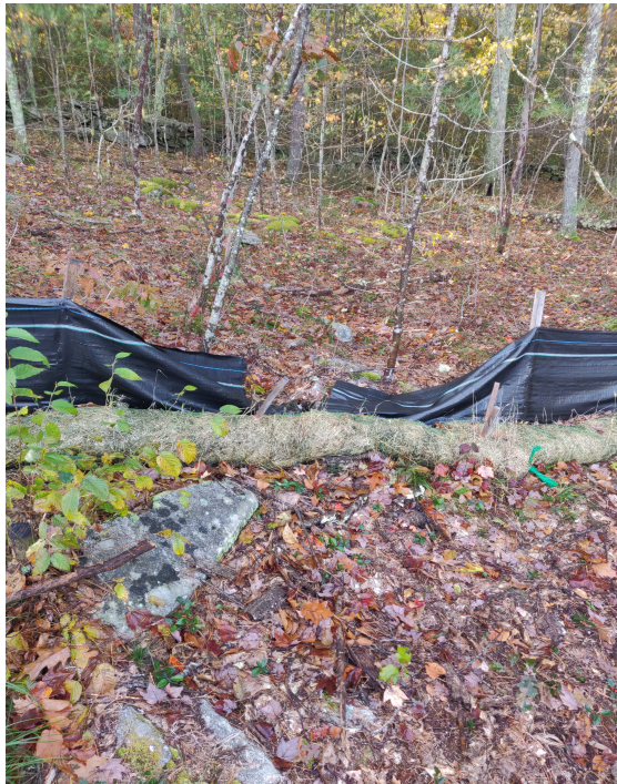
View of the damaged silt fence in southern perimeter of Site —facing south.
