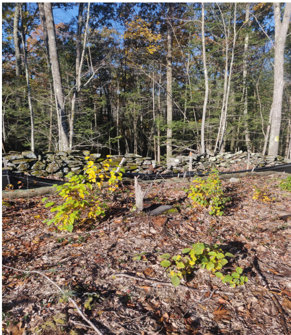
View of damaged silt fence in south west portion of the Site —facing south west
