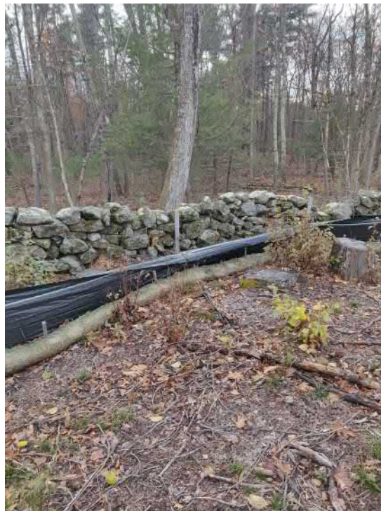
View of damaged silt fence in south west portion of the Site —facing south west
