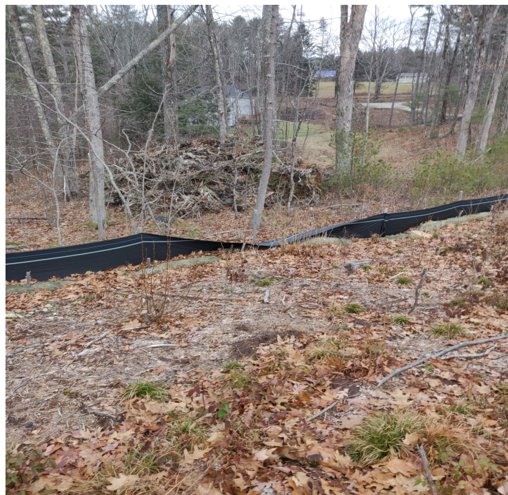
View of damaged silt fence in north western portion of the Site —facing north west
