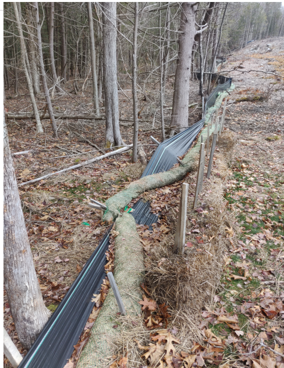
View of area downgradient of Discharge 2—facing north west.
