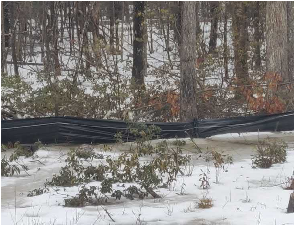
Photo 4 View of the flooded straw wattle and silt fence located up-gradient from Discharge 2 — Facing north west
