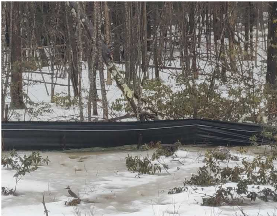
View of the flooded straw wattle and silt fence located up-gradient from Discharge 2 — Facing north west
