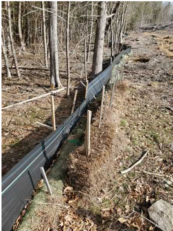
View of area downgradient of Discharge 2—facing north west.
