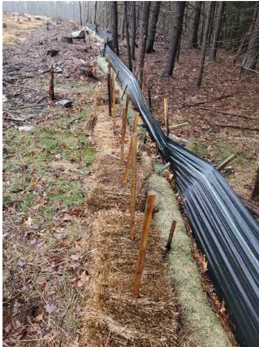
View of area downgradient of Discharge 2—facing south west.
