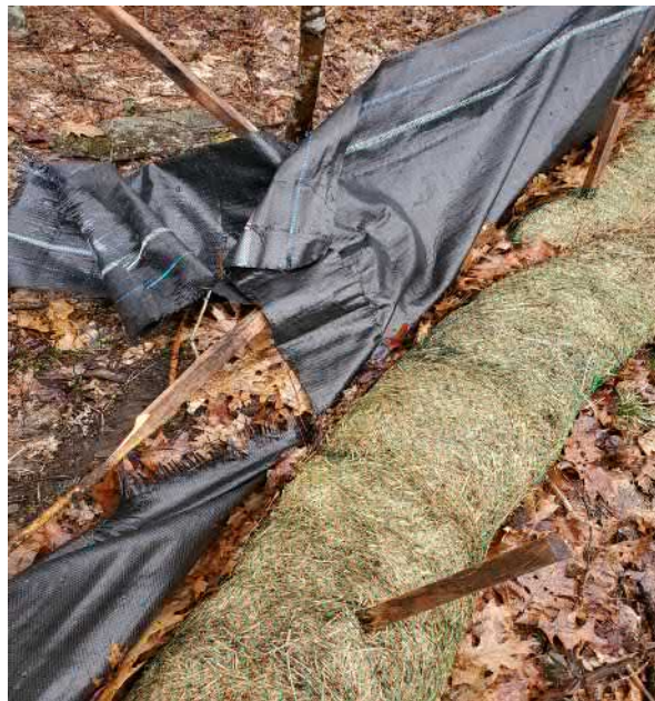
View of damaged silt fence in south east portion of the Site —facing south east
