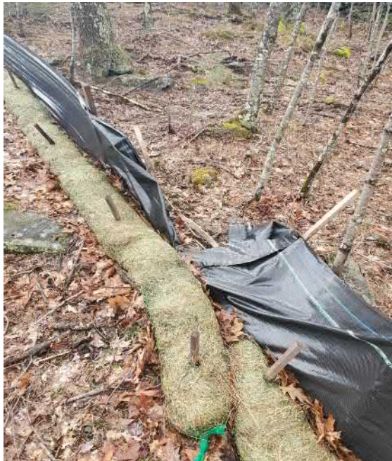
View of damaged silt fence in south east portion of the Site —facing south east
