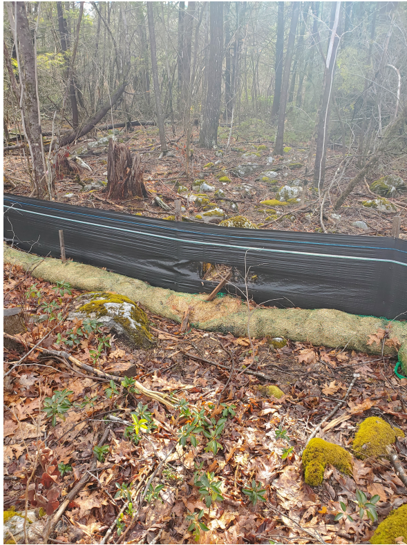
View of damaged silt fence in north east portion of the Site —facing north east
