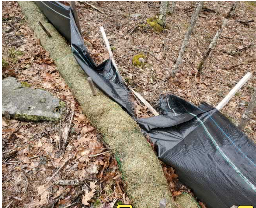
View of damaged silt fence in south east portion of the Site —facing north east
