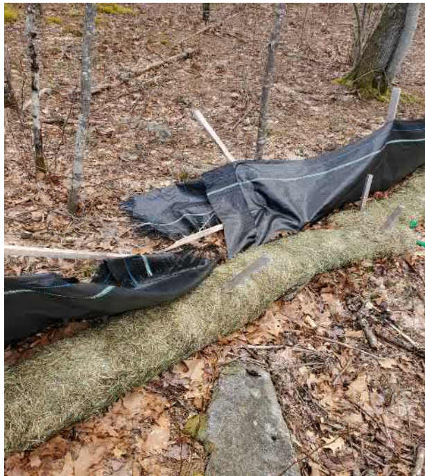
View of damaged silt fence in south east portion of the Site —facing south east
