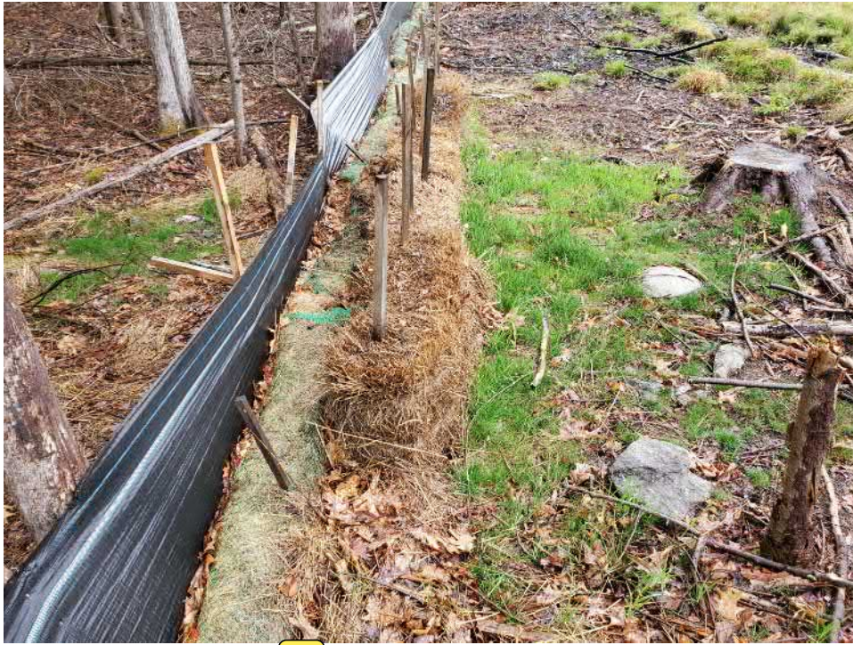
View of seed grass at Discharge 2 — facing north
