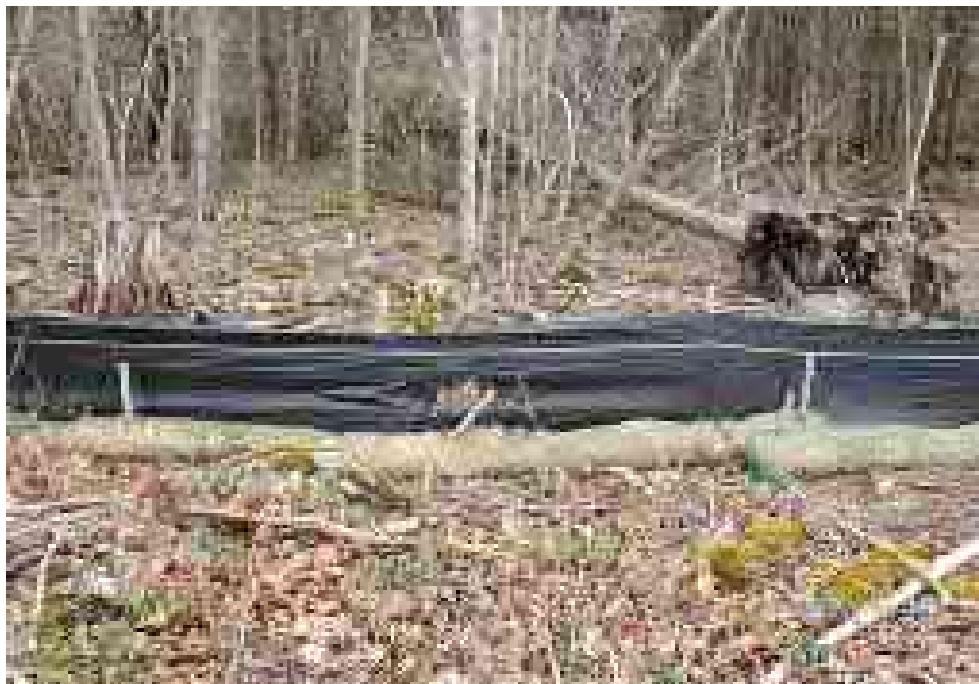
View of damaged silt wattle in north eastern portion of the Site — facing north east
