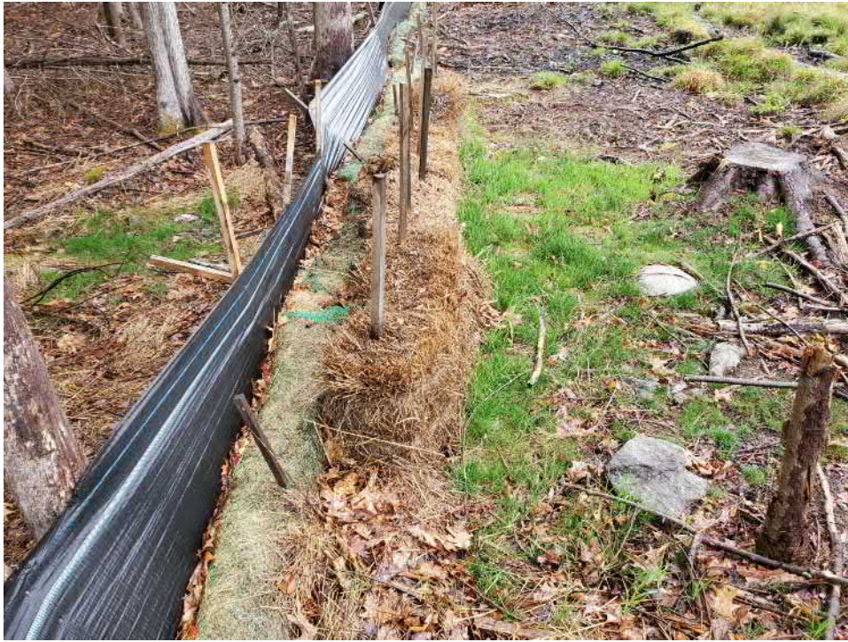
View of seeded grass at Discharge 2 — facing north
