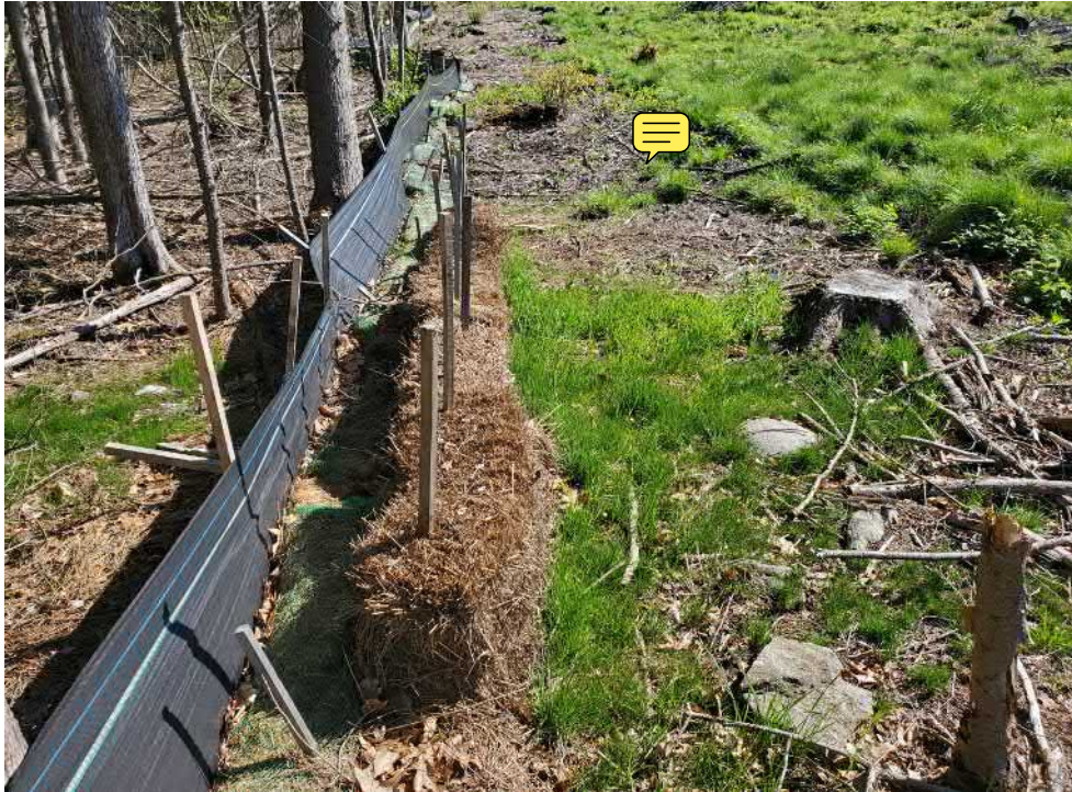
View of silt fence and grass at Discharge 2 — facing north
